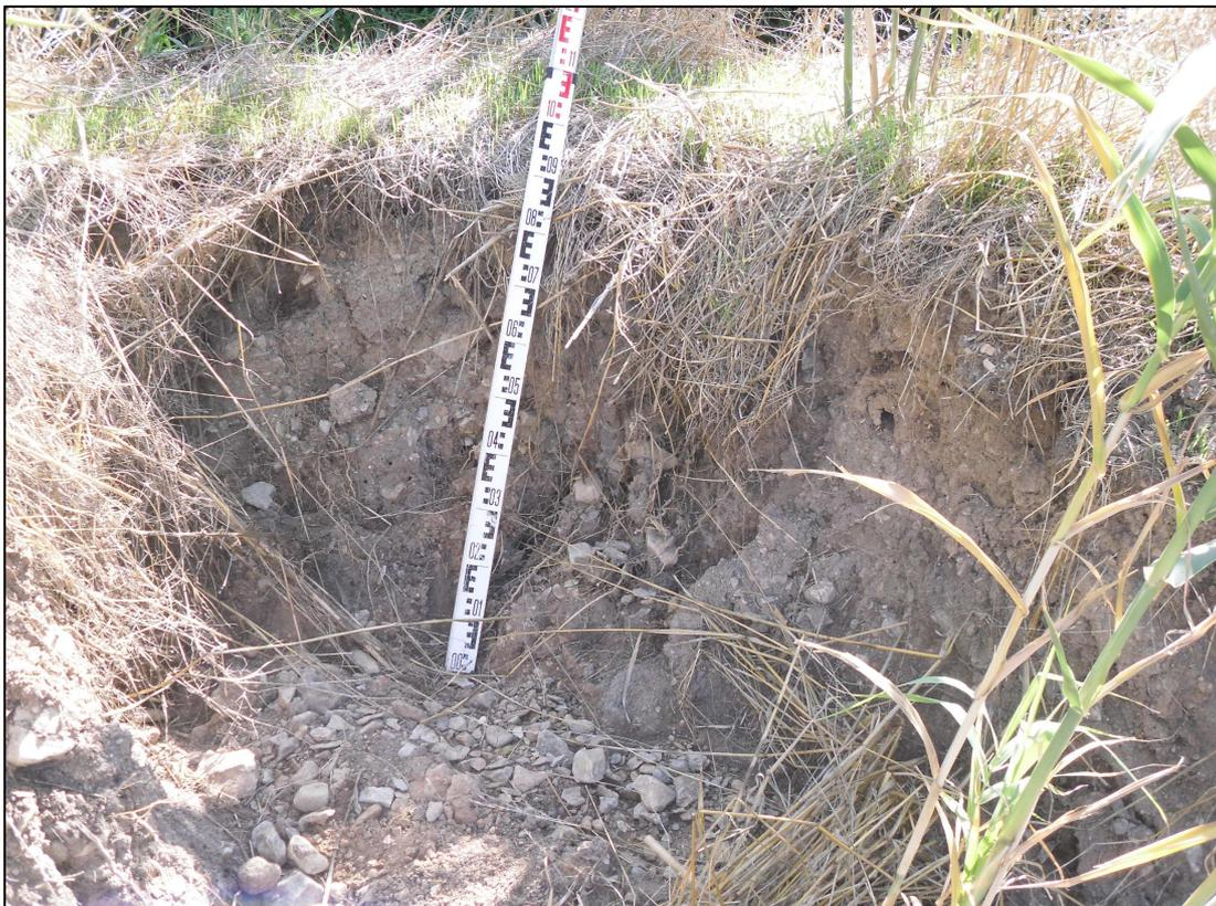
*FIGURE 5 : AMORCE D'EROSION DE LA BERGE RIVE DROITE DU GAUDRE DE LA CROIX AU DROIT DU PROFIL P21*
